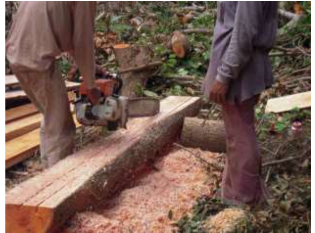
Photo 7 Completing the cut to full depth returning back to the starting point.
